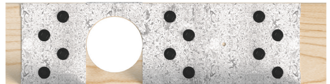
Figure 7: Top Plate Stiffener Installed with Black Screws
