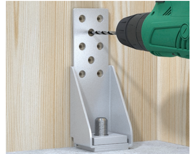
Figure 2 Installation of the Multinail tie-down bracket with washer. Pre-drill for all screws using a 5.0mm diameter drill bit
