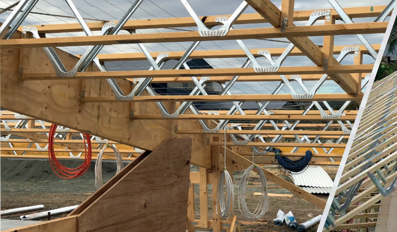
▼ Curved roof trusses
