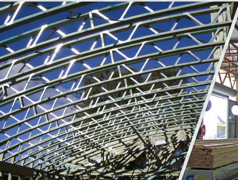
▼ Curved roof trusses
