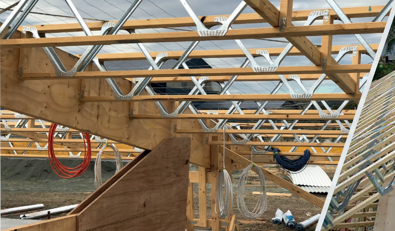
▼ Curved roof trusses
