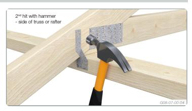
1. Place the Truss Fix in position on the top plate (wall) to cover one or two wall plates (whichever is required). Hit Truss Fix teeth into top plate with hammer.
