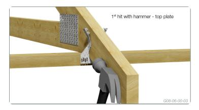
1. Place the Quad Grip in position on the top plate (wall) to cover one or two wall plates (whichever is required). Hit with hammer on one side of the Quad Grip.
